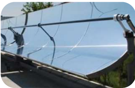
Parabolic trough: curved mirrors that reflect heat
