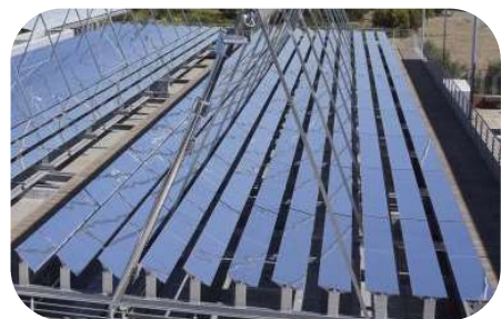
Linear Fresnel: rows of parallel mirrors are angled to reflect
