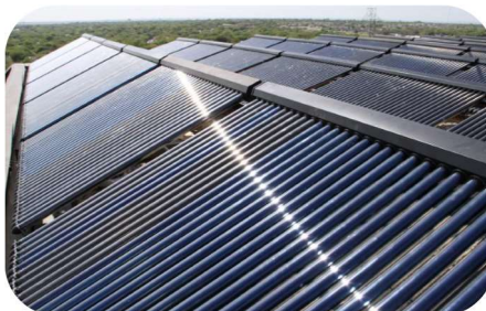
Evacuated tube: closed tubes containing heat transfer liquid
